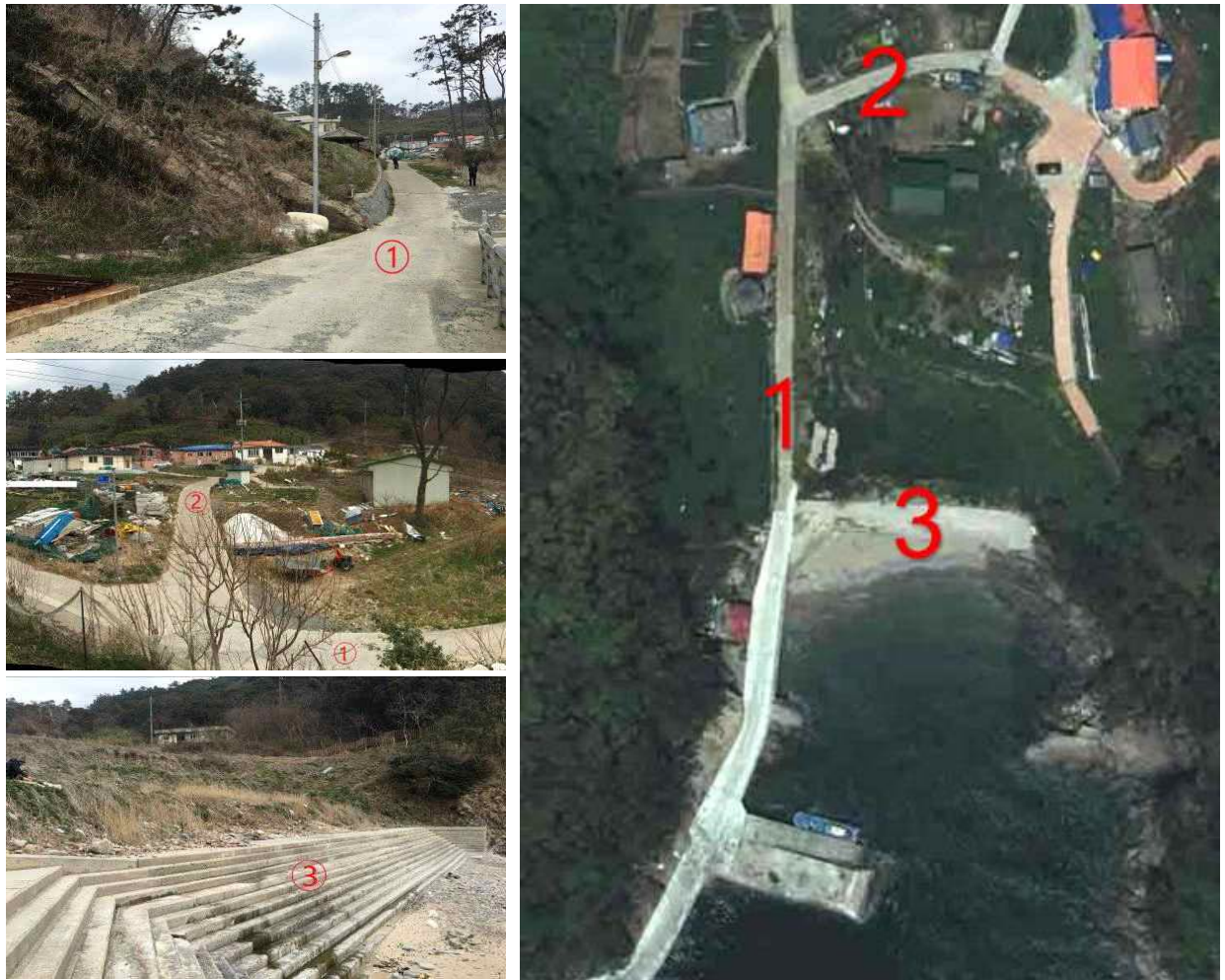
[Fig. 1-4] Facilities to be preserved
